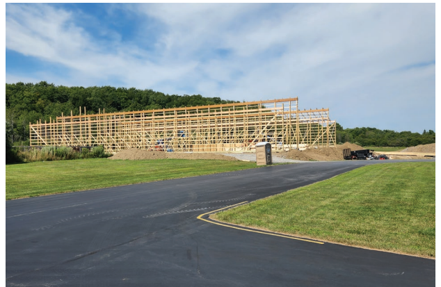
New construction underway at the Park Warner warehouse facility.
